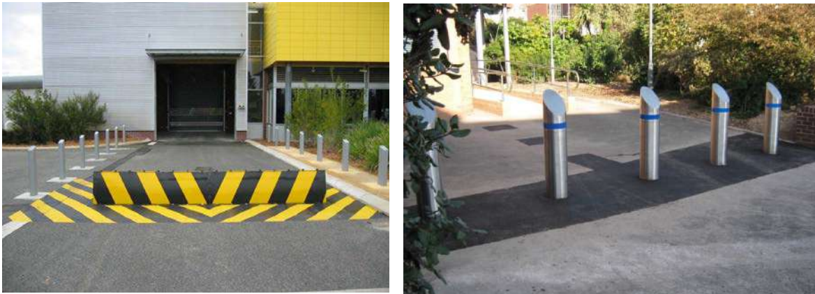
Figure 2 - Anti-RAM Barriers to prevent penetration of vehicles
